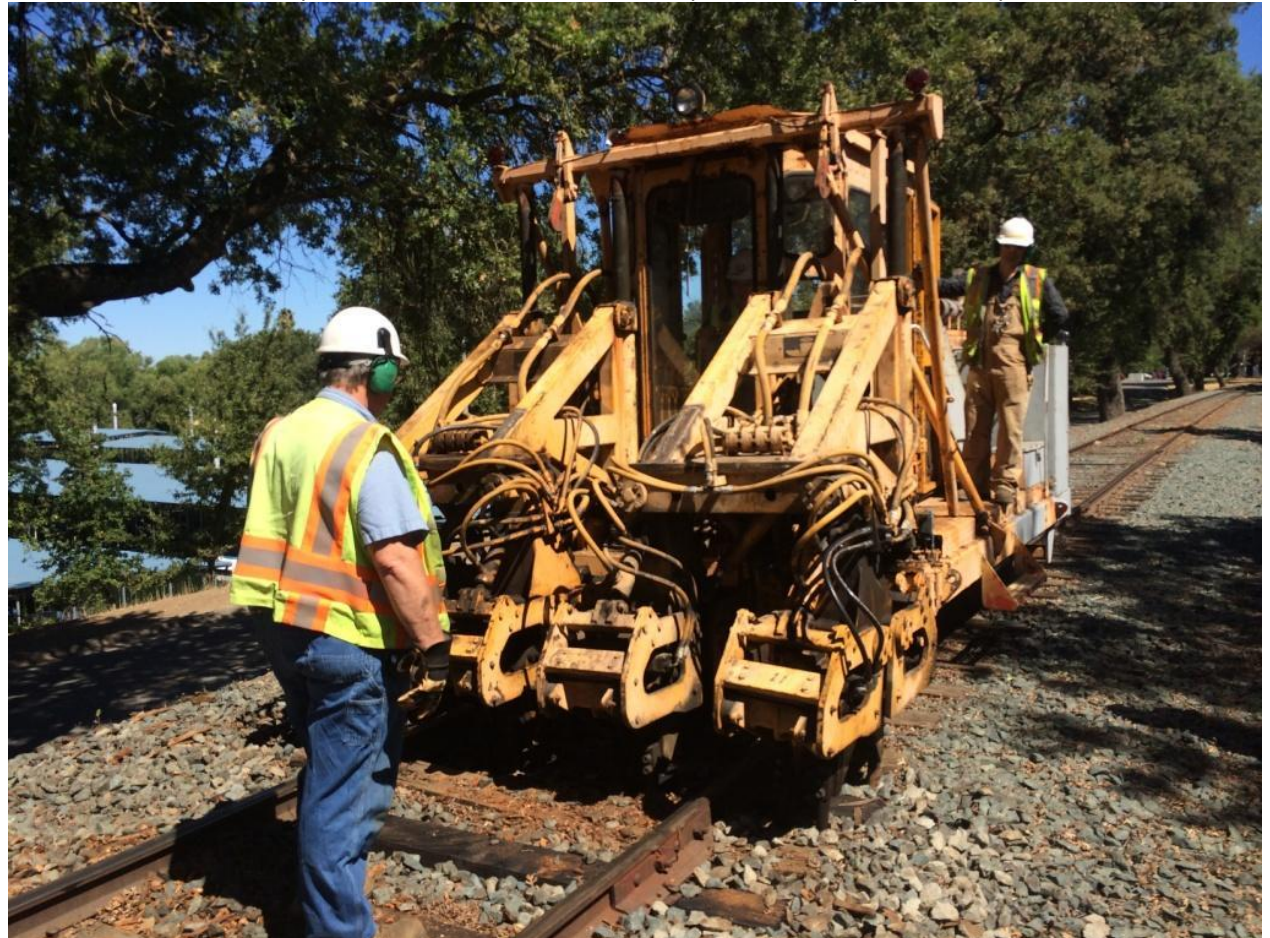
Chris directs Heather in the old-old tamper tamping our newly placed ties
