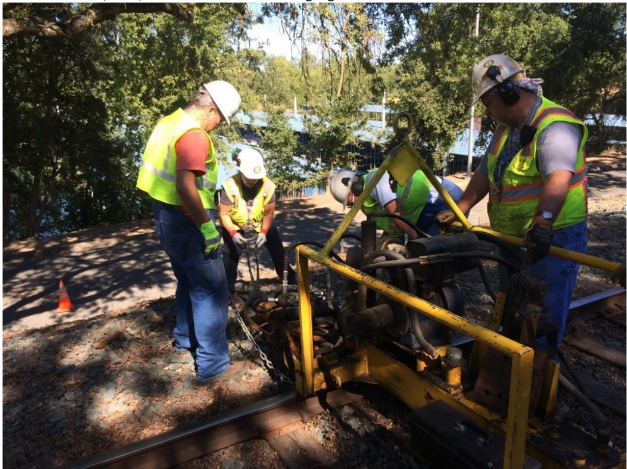
John, Pam, Clem, and Mike F. attempt to pull a rotten tie
