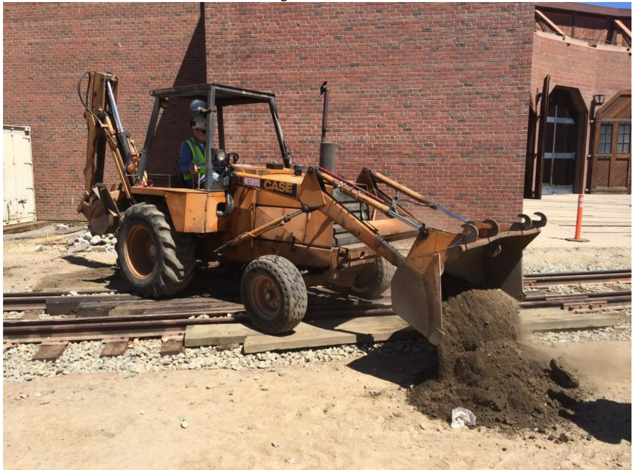
Alan in the back-hoe building the ramp on the west side of the Whisker Track
