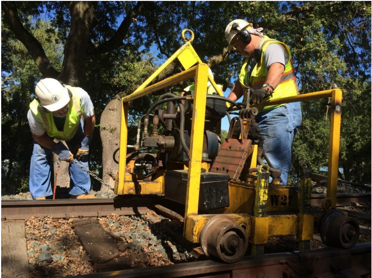
Clem and Mike F. employ chains to pull out a rotten tie
