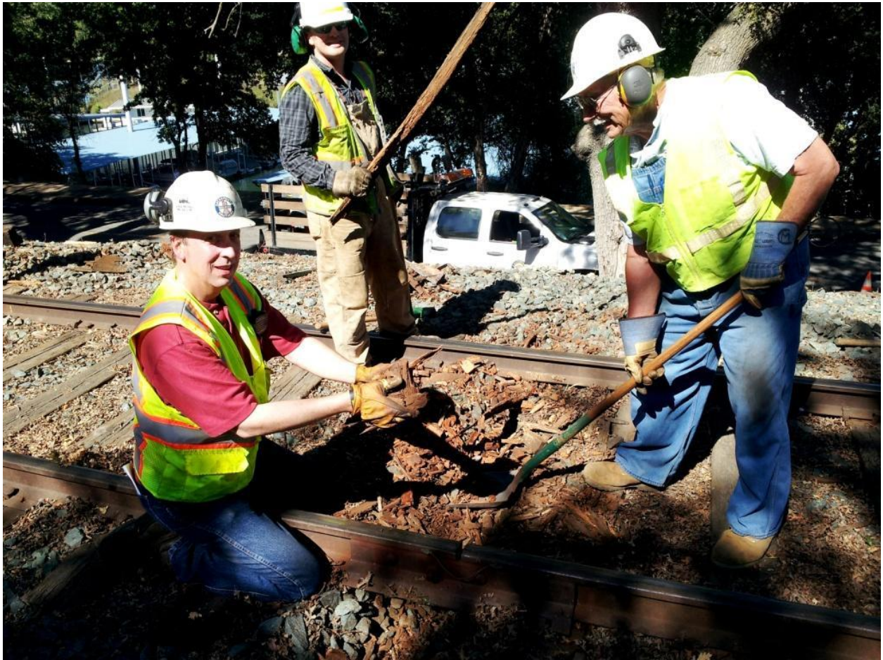
This is a tie?
