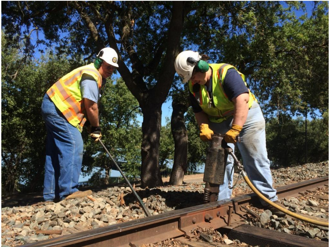
Chris nips the tie as Heather drives the spike with the pneumatic spiker
